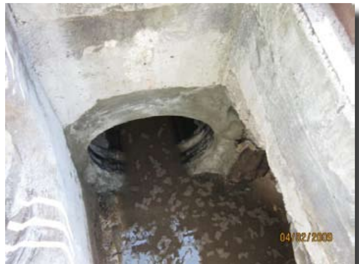
The rehabilitated culvert, with water flowing through.
