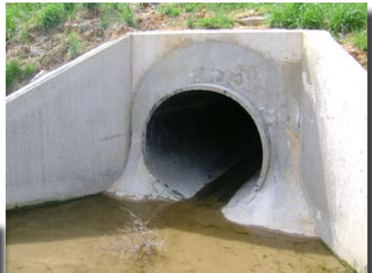
The completely rehabilitated culvert.
