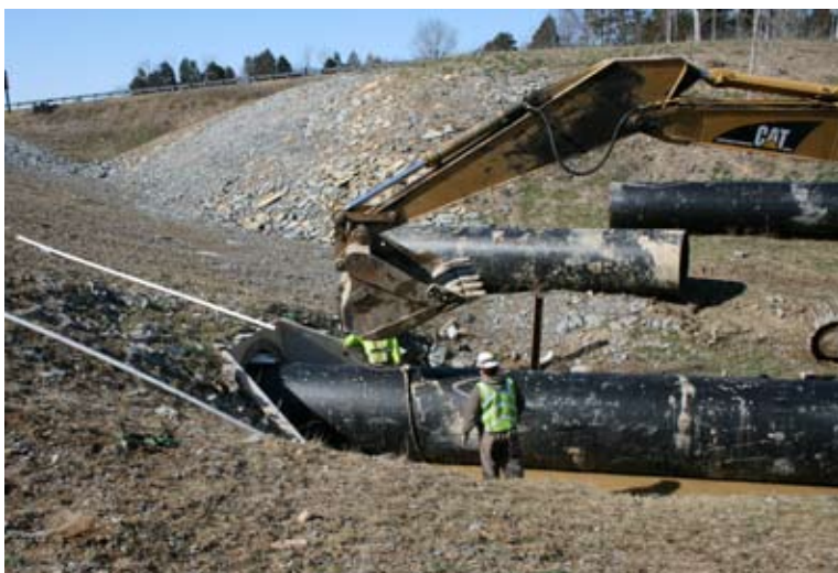
The Snap-Tite installation.
