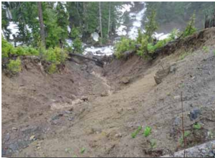
Figure 2: Looking down-slope from the culvert outfall.
