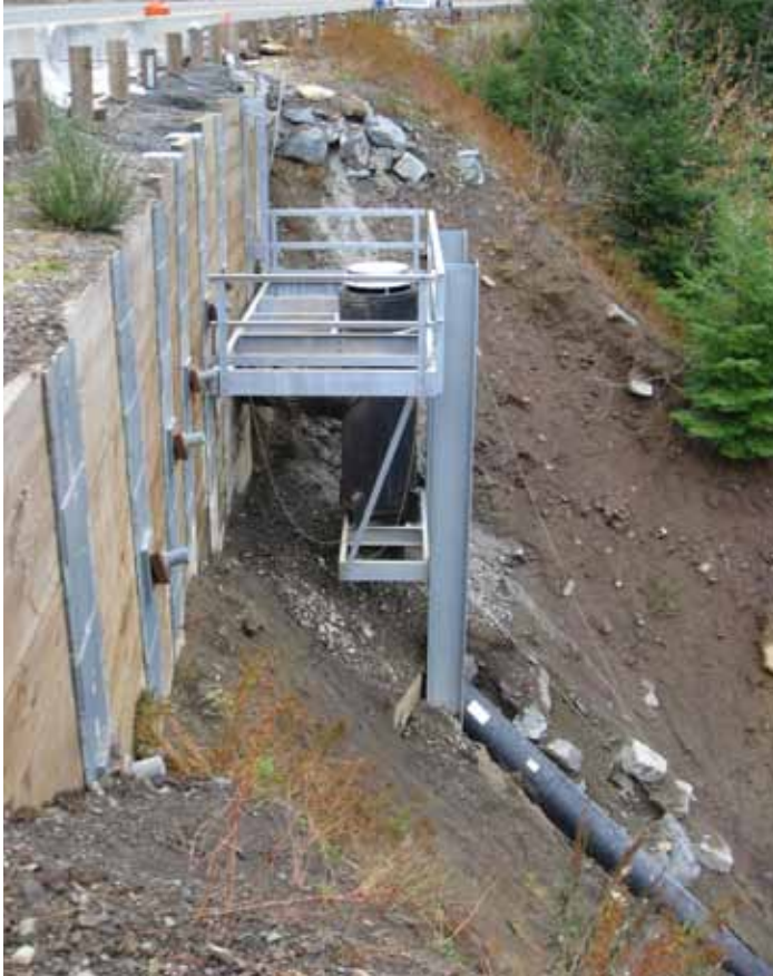
Figure 4: The installation complete.
