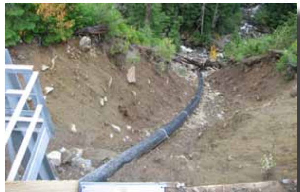
Figure 5: The down-slope pipe.
