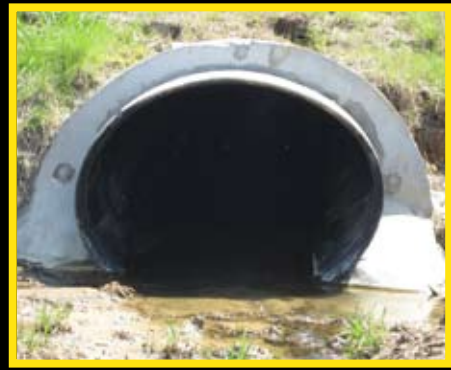
Above: A culvert, rehabilitated with Snap-Tite oval pipe.
