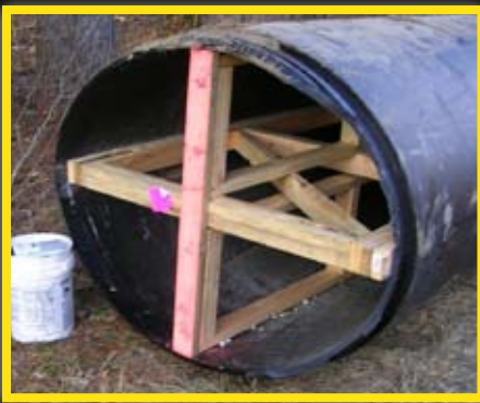
Above: Oval Snap-Tite Pipe with struts inside, before installation.
