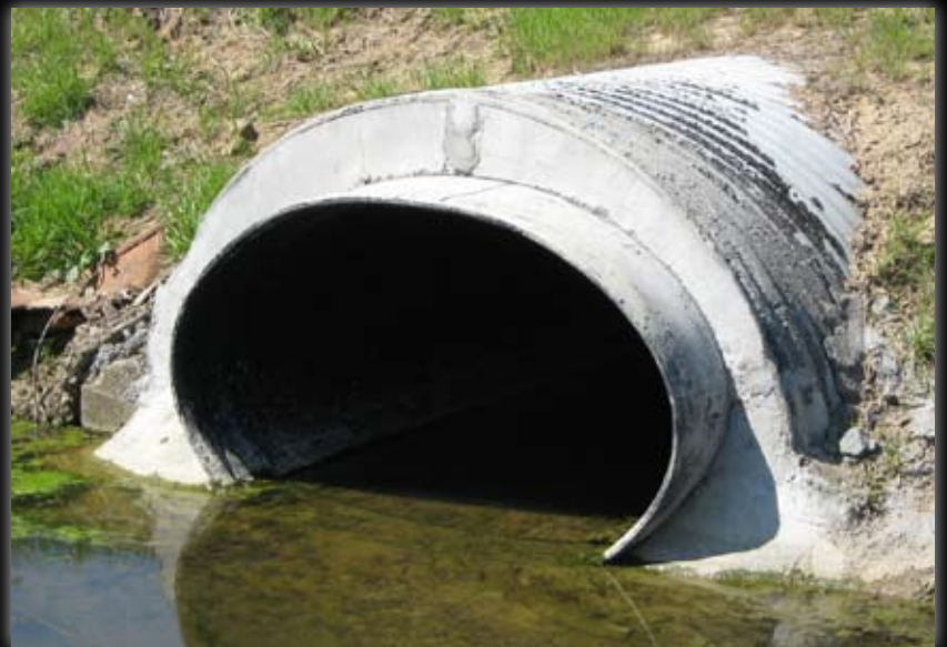
Left: The installation of oval Snap-Tite pipe rehabilitating a failing culvert under a major interstate. Above: A completely rehabbed culvert using Snap-Tite oval pipe.
