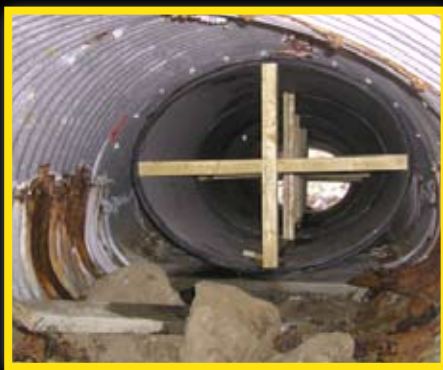
Above: Snap-Tite pipe coming through a deteriorating culvert during installation (struts will be removed once completed).
