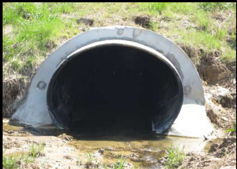
Left: The installation of oval Snap-Tite pipe rehabilitating a failing culvert under a major interstate. Above: A completely rehabbed culvert using Snap-Tite oval pipe.
