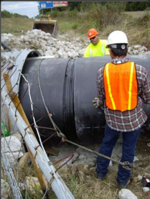
Left: The installation of oval Snap-Tite pipe rehabilitating a failing culvert under a major interstate. Above: A completely rehabbed culvert using Snap-Tite oval pipe.
