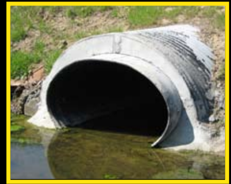
Above: A culvert, rehabilitated with Snap-Tite oval pipe.
